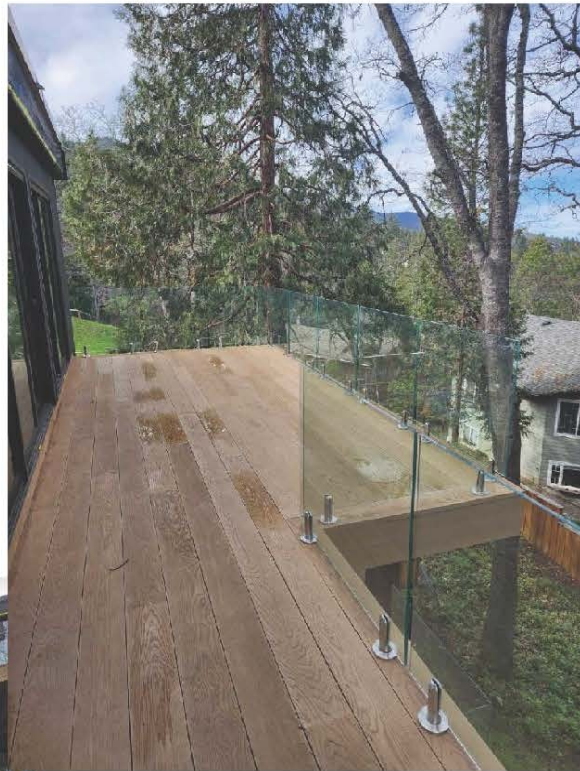
1/2" Clear Tempered Glass Railing
