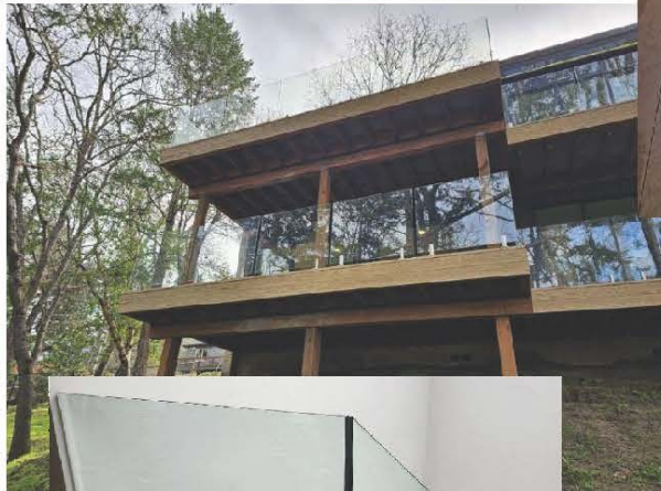
1/2" Clear Tempered Glass Railing
