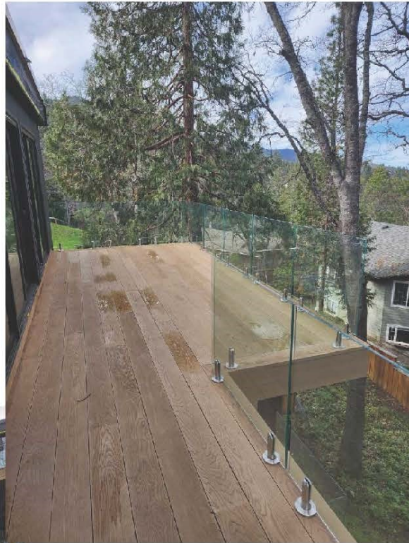
1/2" Clear Tempered Glass Railing
