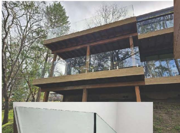
1/2" Clear Tempered Glass Railing
