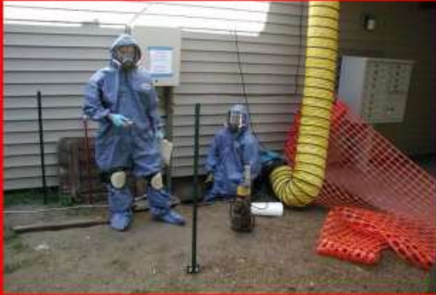
Residential & Commercial Testing / Abatements
