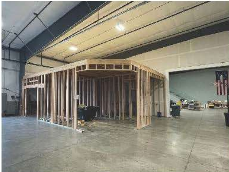
SOGAM New Office Expansion
