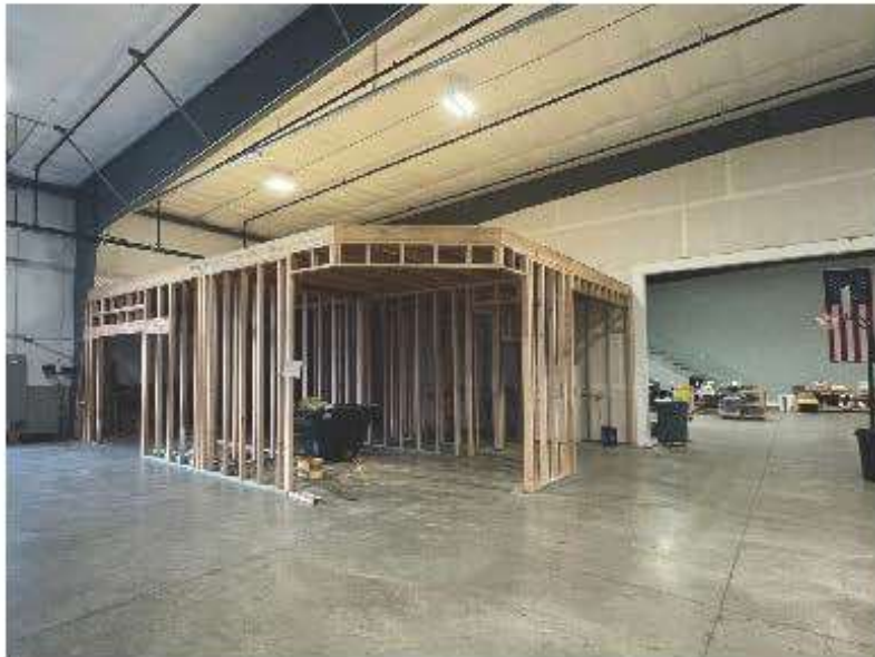
SOGAM New Office Expansion
