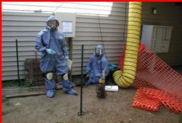
Residential & Commercial Testing / Abatements
